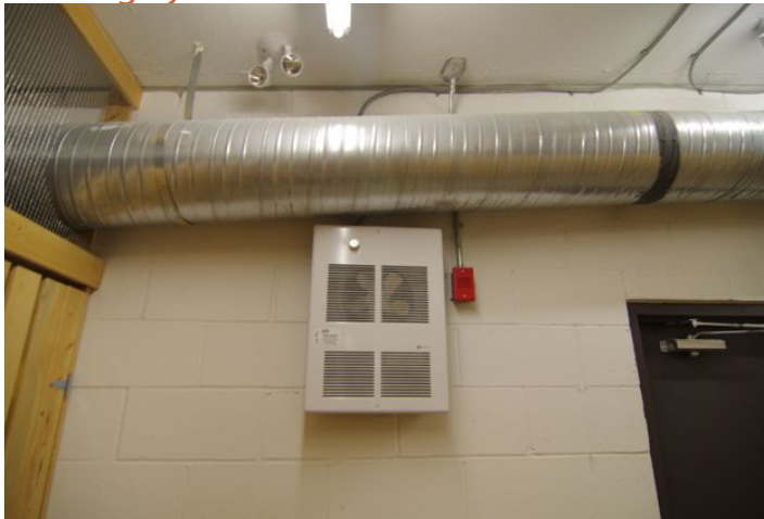
Photo 5.6— Force flow unit heater in storage room
