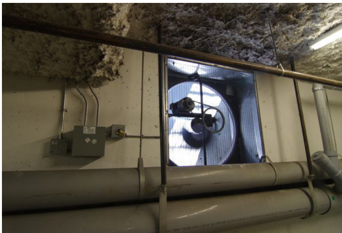
Photo 5.9—Sidewall exhaust fan in parking garage.
