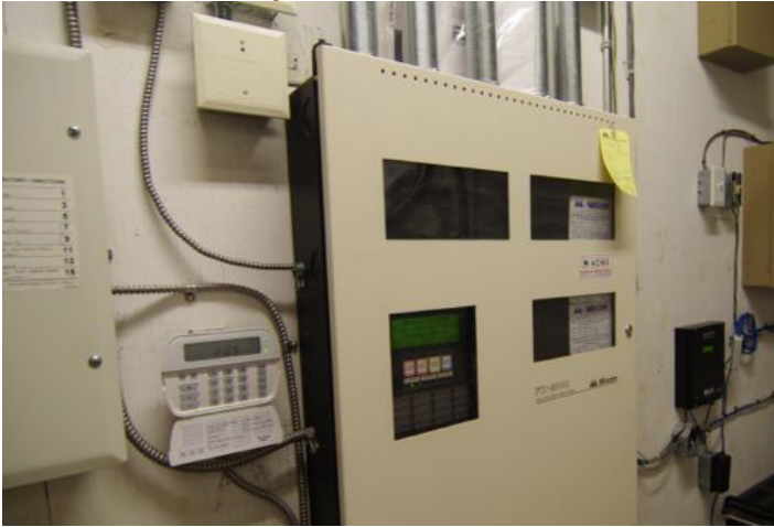
Photo 7.2-- Main Fire Alarm Control Panel in Communication Room
