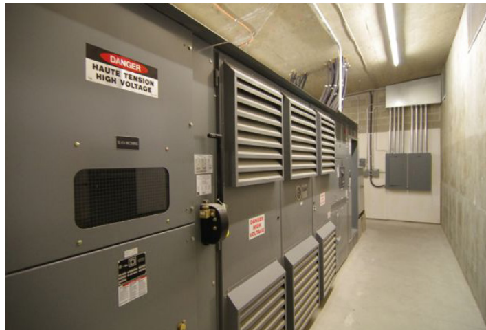
Photo 6.1— Load break switch, main transformer and Central Distribution Panel in electrical room.
