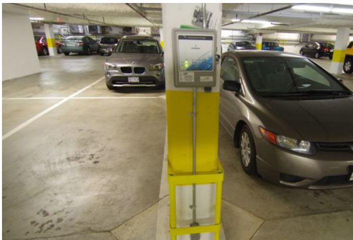
Photo 5.10— Gas detection system mounted on column in parking garage.
