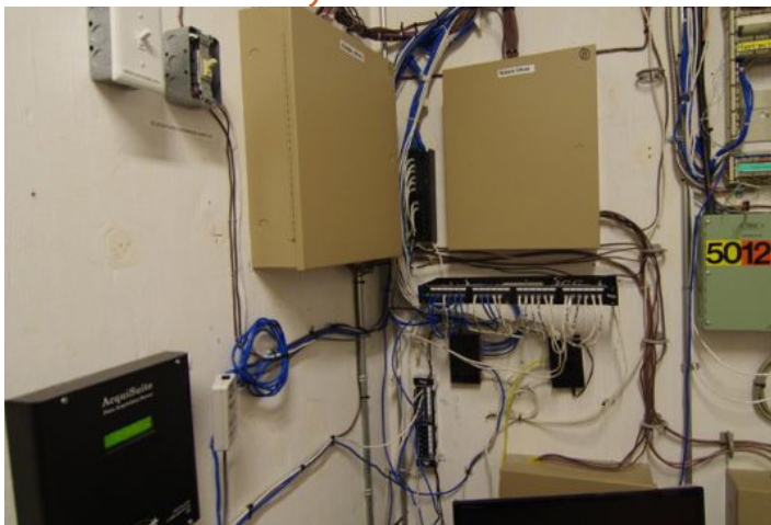
Photo 6.7— Fibre optic demarcation cabinet and cable systems
