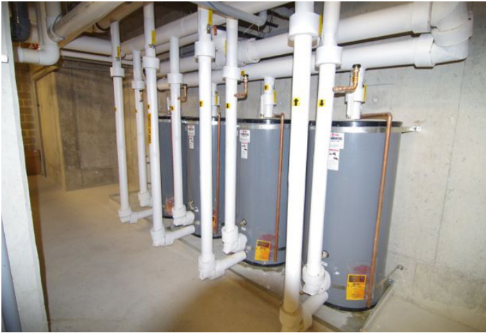
Photo 5.3 — Main domestic hot water storage tanks and expansion tank. Temperature noted to be 135°F.
