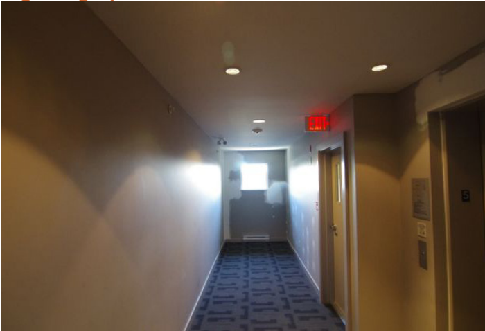
Photo 6.2— Hallway lights in interior of residential building (compact fluorescent pot lights) and MR-16 pot lights.
