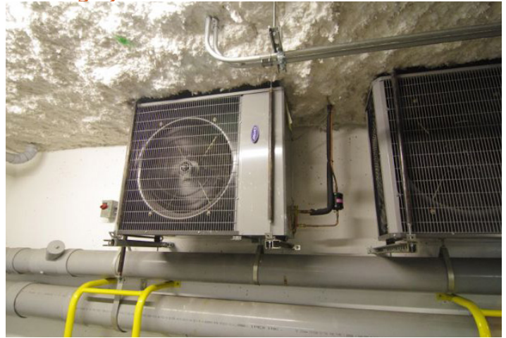
Photo 5.7— An air cooled condensing unit in parking garage serving the commercial units. The hot gas and liquid lines run across the ceiling of the parking garage to the fan coil units.
