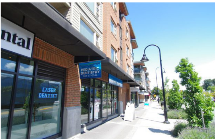
Photo 1.2—Elevation showing commercial suites on Marine Drive
