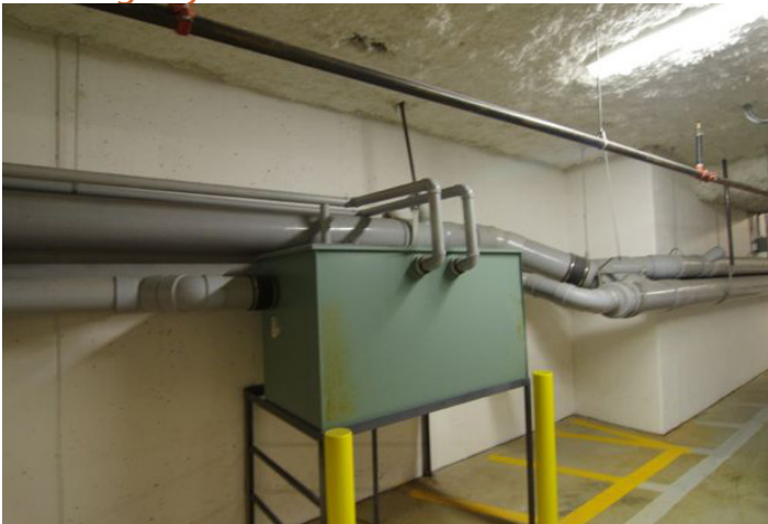
Photo 5.4— Interceptor on storm drainage system in parking garage
