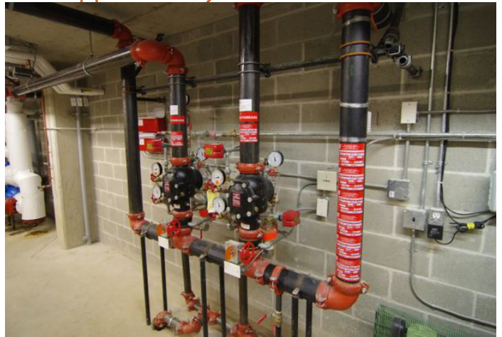
Photo 7.1— Dry valve and flow switch on fire suppression system
