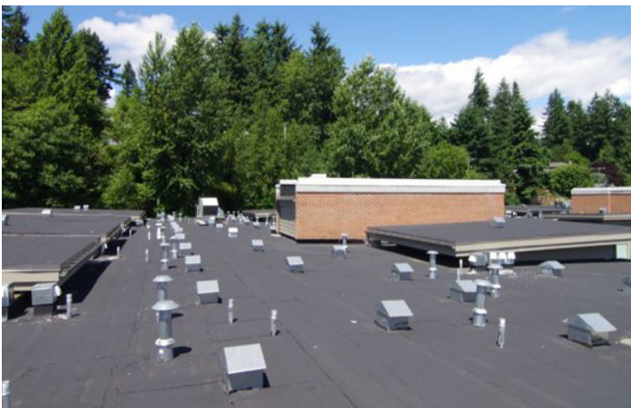
Photo 1.1—Roof level view looking north
