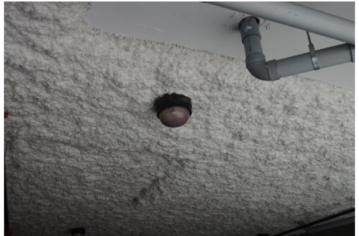
Photo D -- Problems with light fixtures throughout building. Lamps are failing far too frequently.
