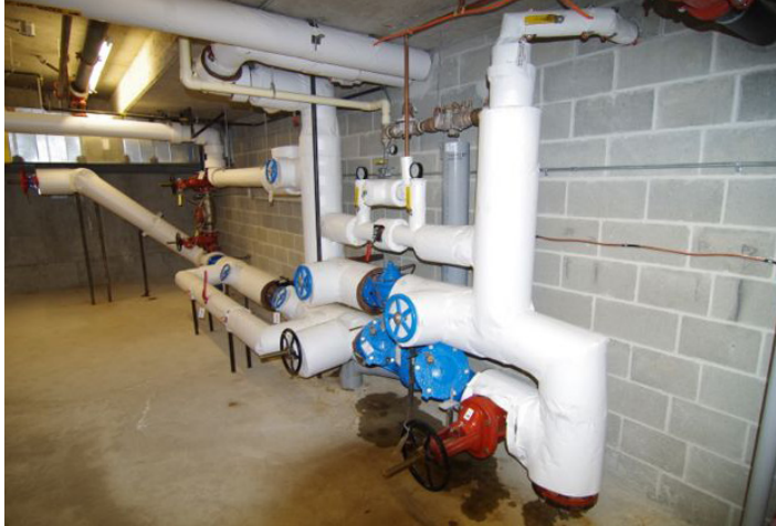
Photo 5.1 — Main domestic water line showing the pressure reducing valves on water supply and the backflow preventers. The incoming pressure is 110 psi and the supply pressure to building is 50 psi.
