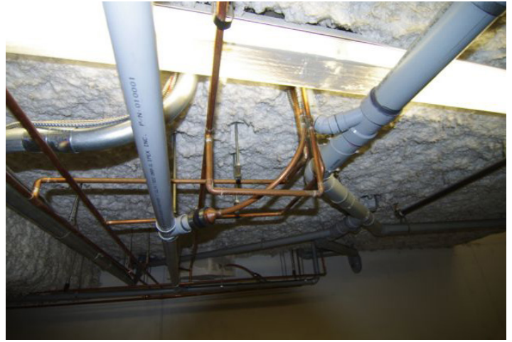
Photo B -- What appears to be un-insulated copper piping for trap primers at the entrance to the parking garage..
