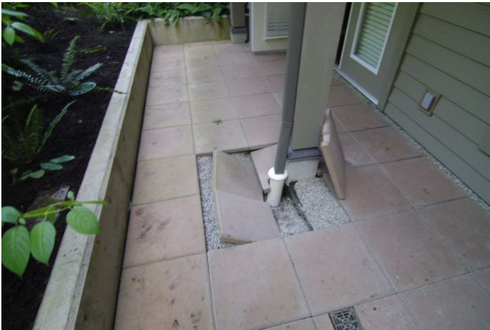
Photo C -- Soil erosion around storm drain on amenity patio area.
