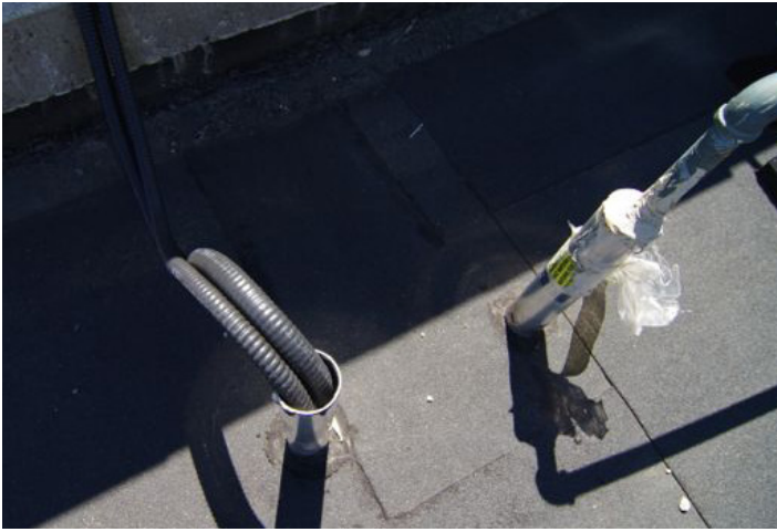
Photo A -- Make-up Air Unit mounted on roof. Note the lack of caulking at roof penetration for electrical wiring.
