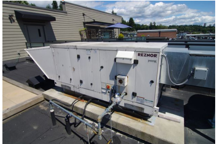
Photo 5.8— Roof mounted make-up air unit.
