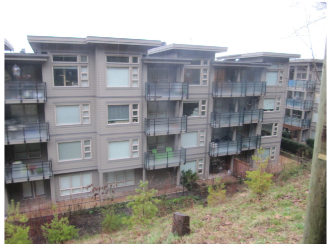
Fig. 1.6.4 North elevation of 1679 Lloyd Ave.
