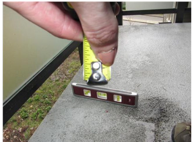
Fig. 4.3.5 Backslope of balcony surface at suite 506, 1679 Lloyd.
