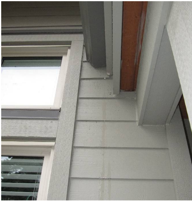
Fig. 4.3.6 Water draining onto wall assembly from balcony gutter above.
