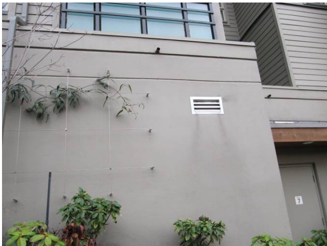
Fig. 3.3.1 A section of coated architectural concrete wall at the first floor.
