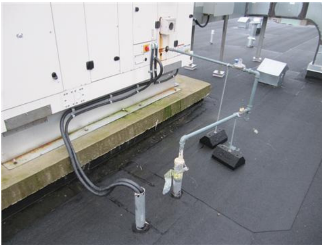
Fig. 4.3.2 Improperly sealed electrical penetrations at roof level.
