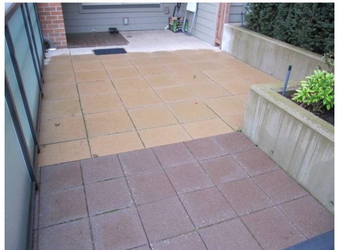
Fig. 3.3.6 Deck at second floor above parkade.
