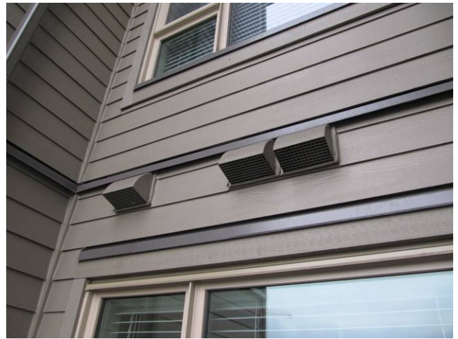
Fig. 4.1.1 Typical exhaust vents at exterior walls.
