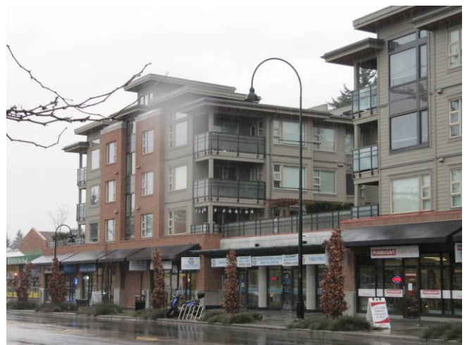
Fig. 1.6.5 Southeast corner of 1677 Lloyd Ave.
