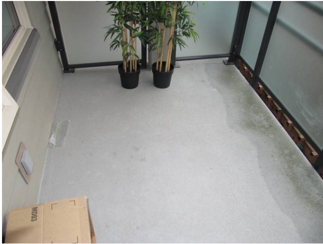
Fig. 3.3.5 Typical balcony with liquid-applied urethane membrane.
