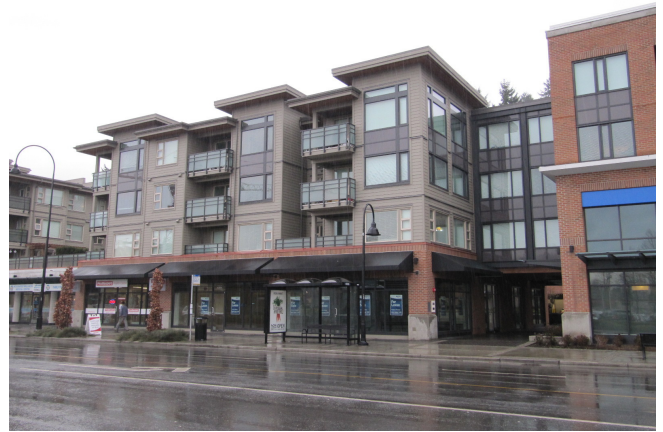
Fig. 1.6.3 South elevation of 1673 Lloyd Ave along Marine Drive.
