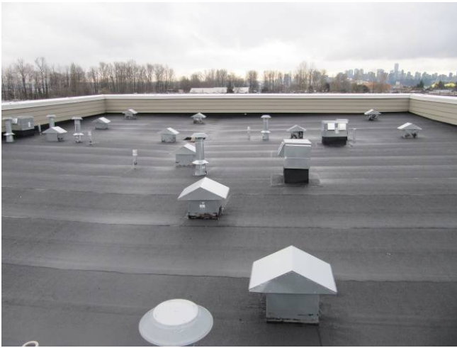
Fig. 4.1.3 Exhaust vents at main roof.
