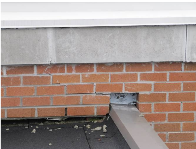
Fig. 4.3.3 Loose bricks and cracked mortar joints at roof level.
