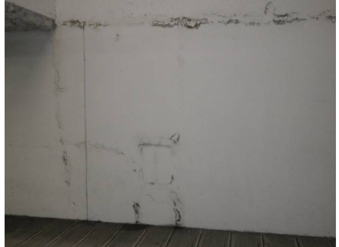
Fig. 4.3.7 Water ingress along entry ramp exterior wall.
