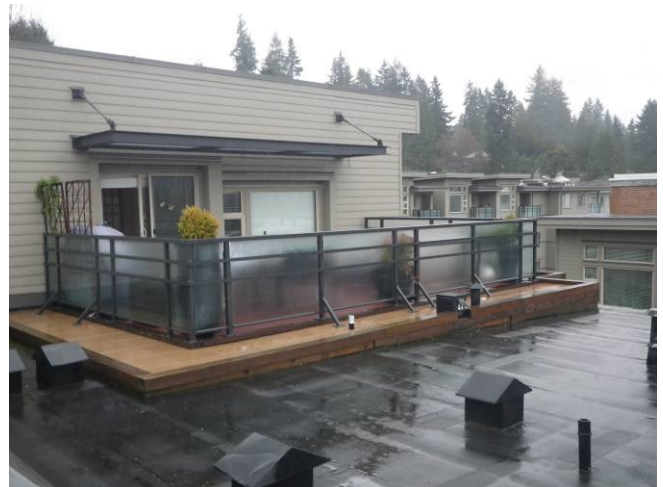
Fig. 3.3.7 Roof deck at fifth floor, 1677 Lloyd.
