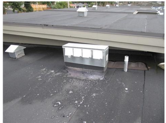
Fig. 4.3.1 Lint accumulation below dryer vents at roof level.
