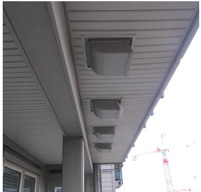
Fig. 4.1.2 Typical exhaust vents at balcony soffits.
